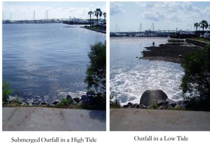
**Figure 2.** Effect of high tides on storm water outfalls (Adapted from Kirk, 2010)
